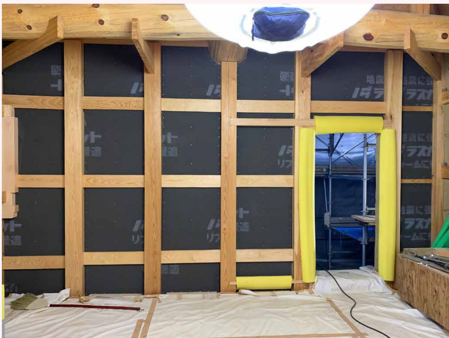
Structural Plywood Installed in the Wall
