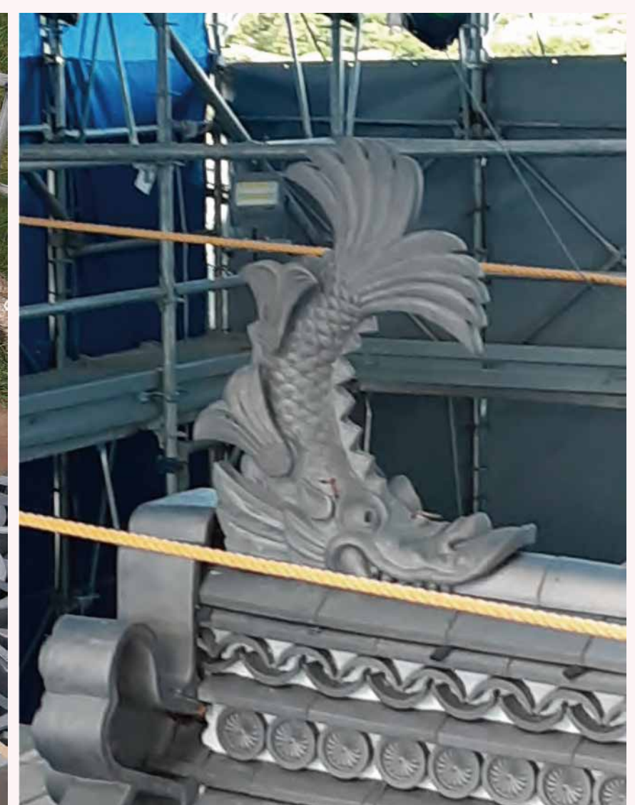
Shachi-gawara on the Roof
