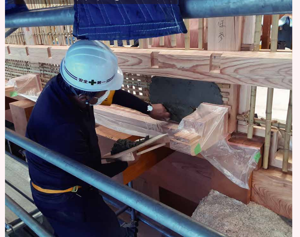
Plasterer Applying Wall Soil
