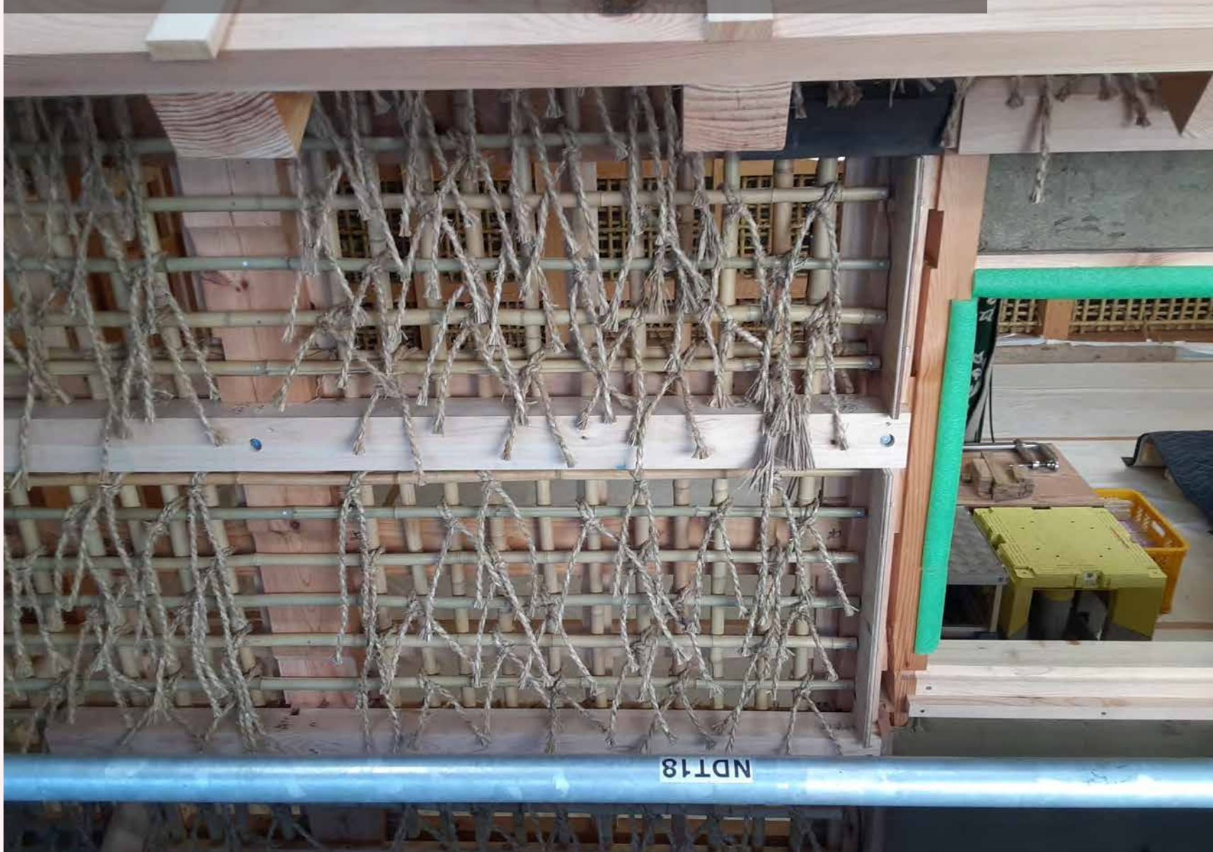
Wall Soil Applied and Waiting to Dry
