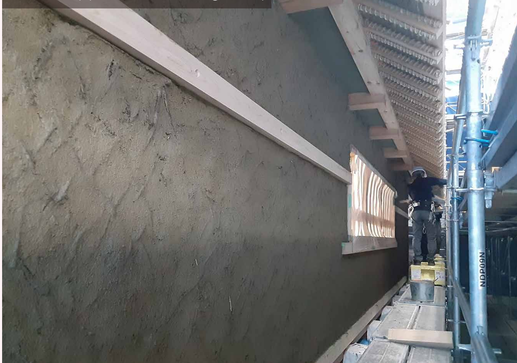
Wall Soil Applied and Waiting to Dry
