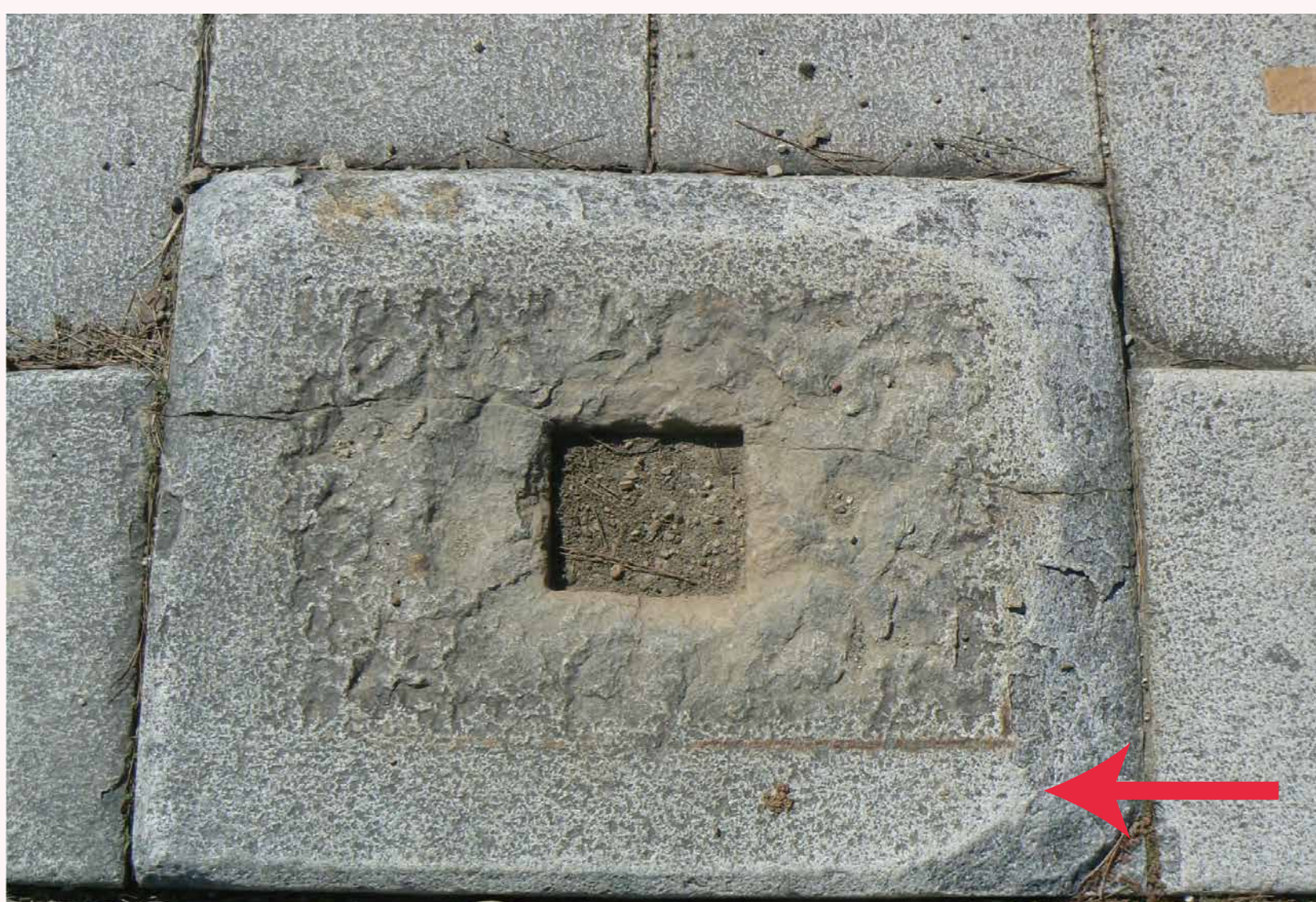
Traces of Column on Foundation Stone (Rust of metal hardware wrapped around the base)
