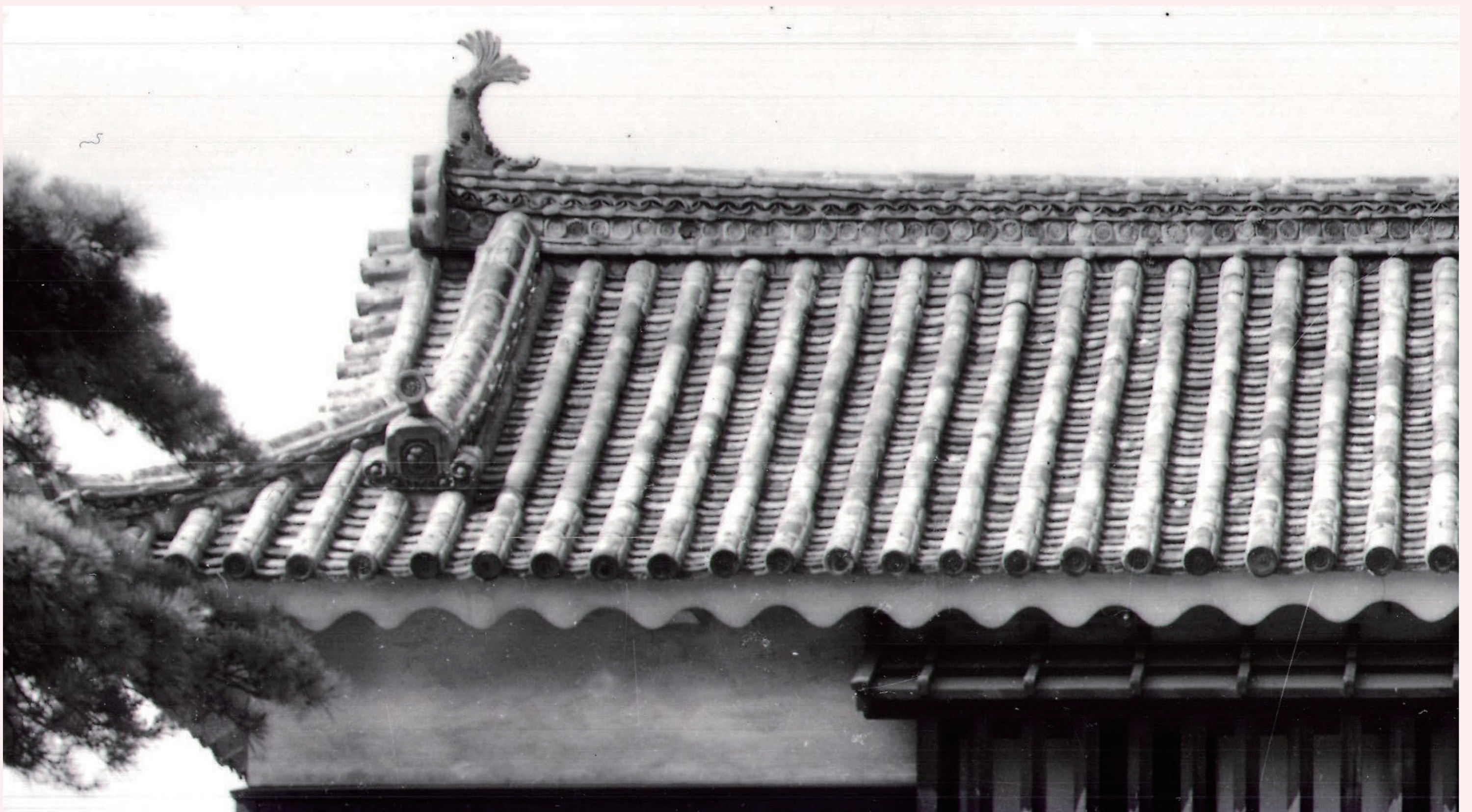
Shape of the Roof Seen on Old Photograph (Courtesy of the Nara National Research Institute for Cultural Properties, Enlarged)
