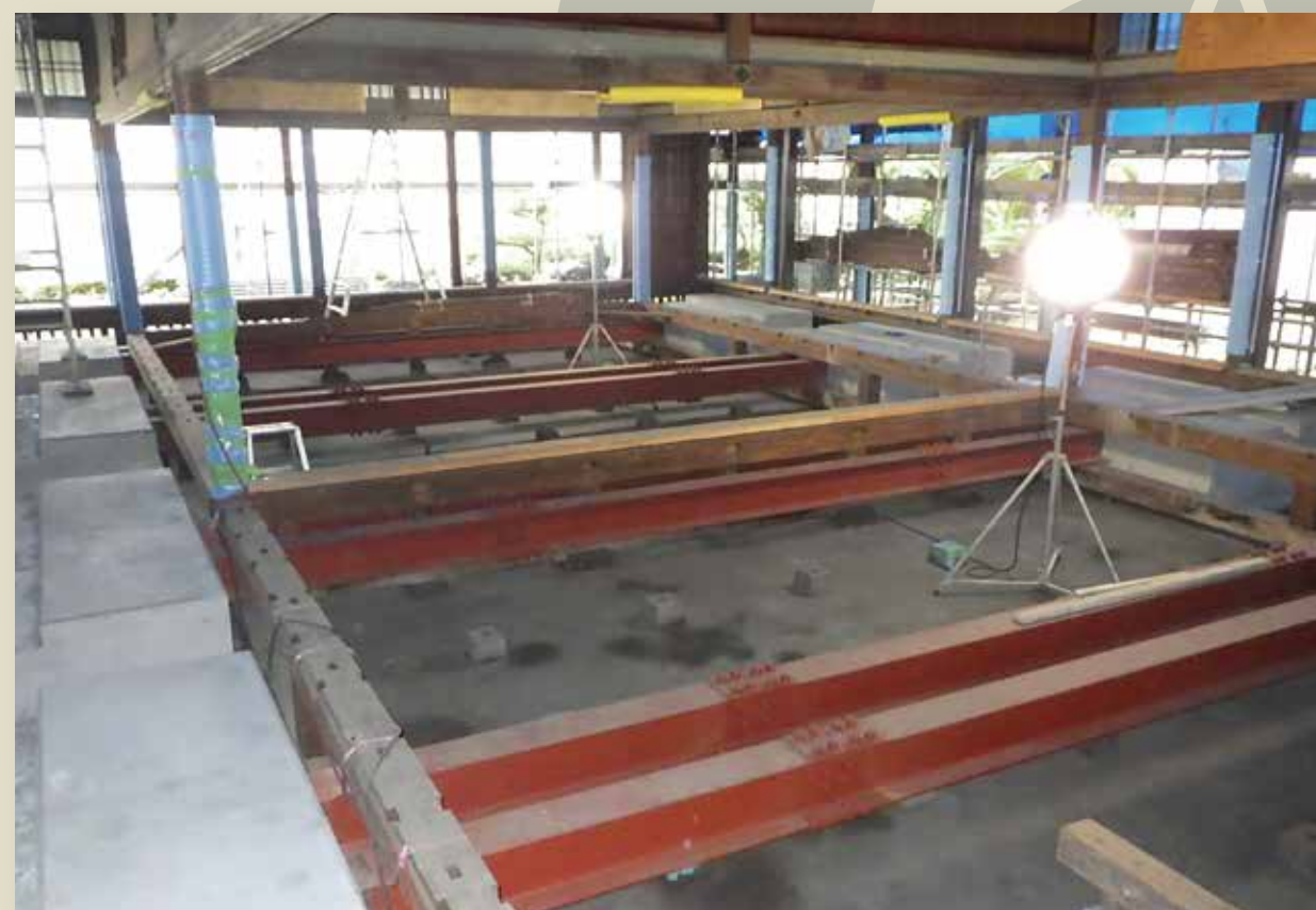
■ Seismic Reinforcement of the Hiunkaku Sotetsu no Ma [cycad room]
