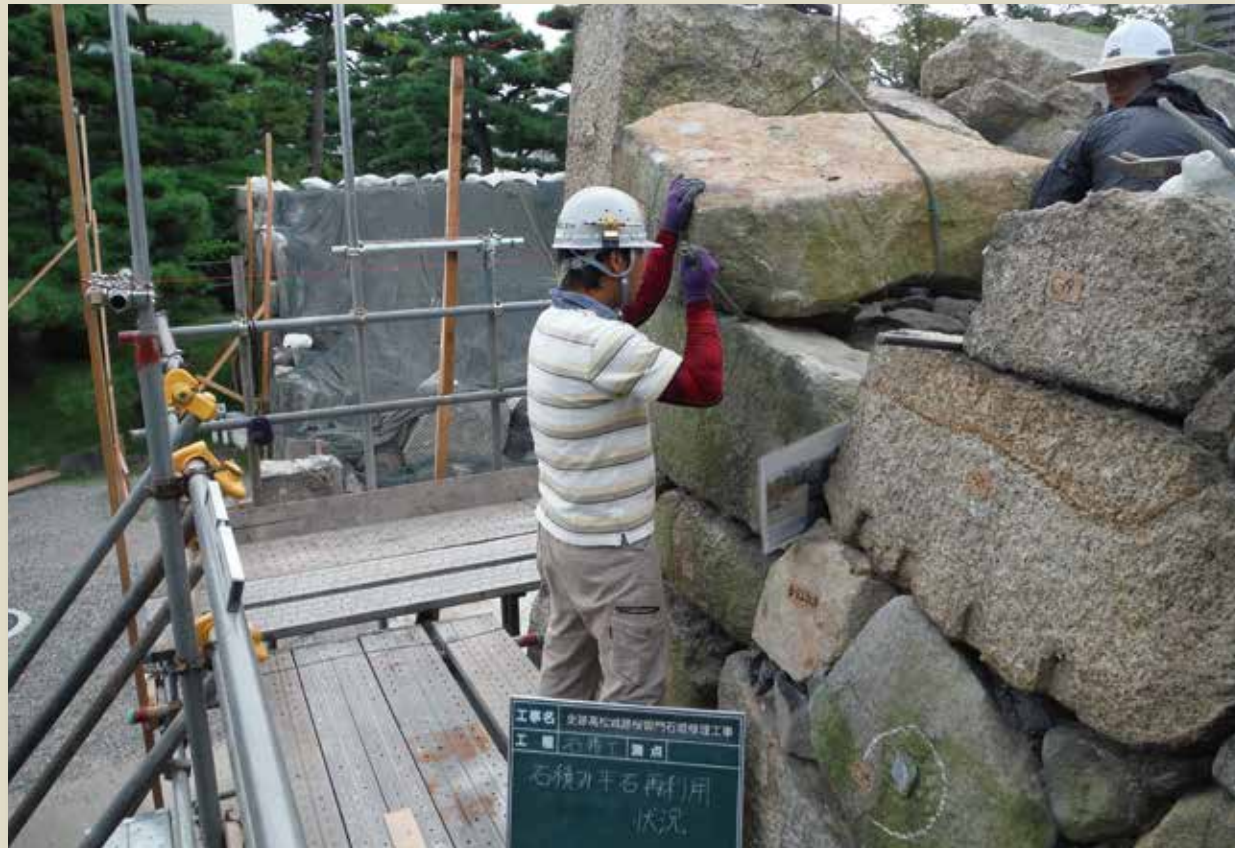
■ Dismantling and Restoration of the Stone Walls
