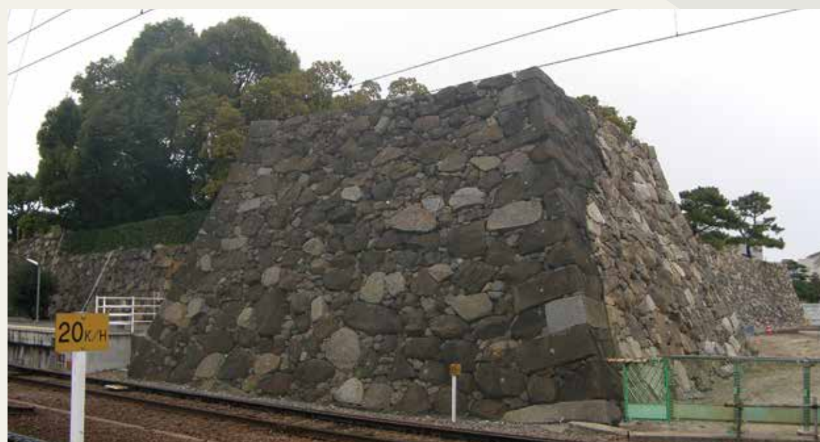
■ Stone Walls Built by the Ikoma Family (foundation of Chikyū Yagura [eternal prosperity tower])
