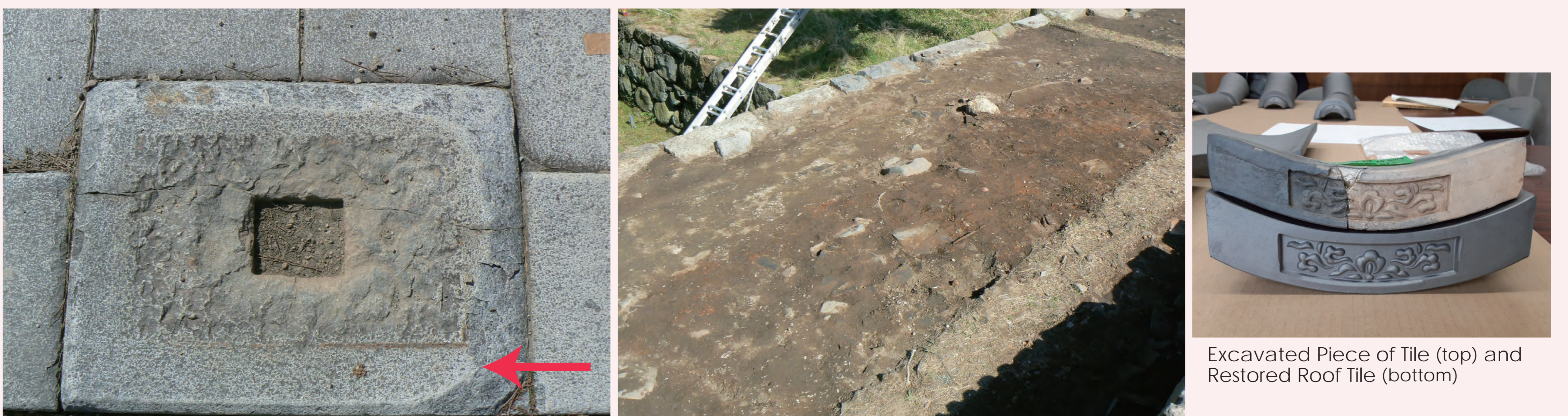
Traces of Column on Foundation Stone (Rust of metal hardware wrapped around the base)
