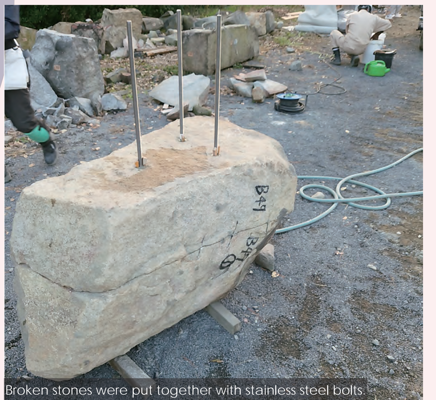
Cracks were reinforced with stainless steel U-pins.
